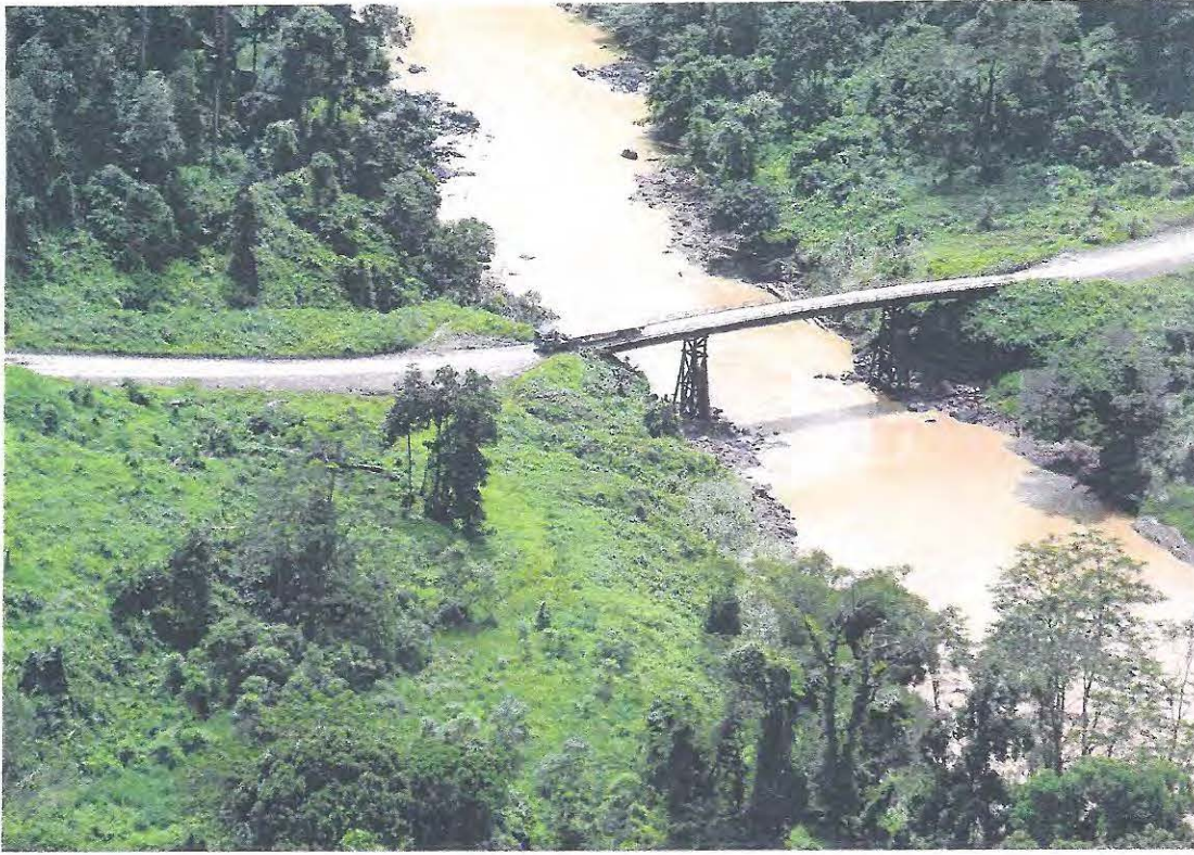
Plate 3: A steel bridge crosses the Kuamut River into Compartment # 1. A riparian reserve of 100 m has been demarcated along the Kuamut River. No logging is allowed within this area.
